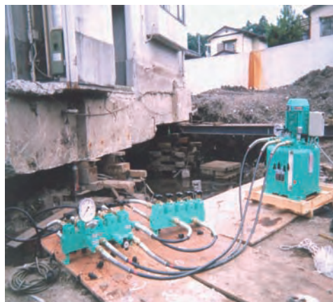
[Up and down of house] Features: Synchronization control under different jack loads
